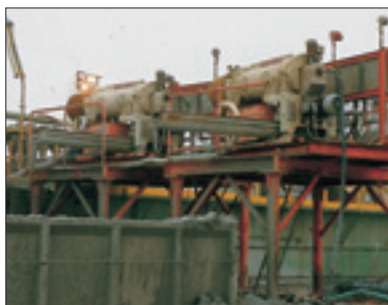
Drilling mud recovery
